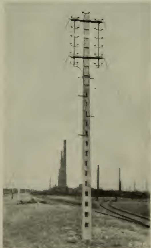
LINE OF REINFORCED CONCRETE TELEGRAPH POLES CARRYING TWENTY-TWO WIRES.
